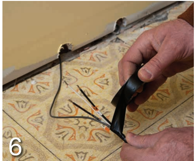
6 Pull the heat-mat leads and the heat-sensor wire through separate conduits.
