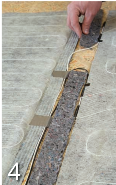
4 Place underlayment in the gaps between heating mats.
