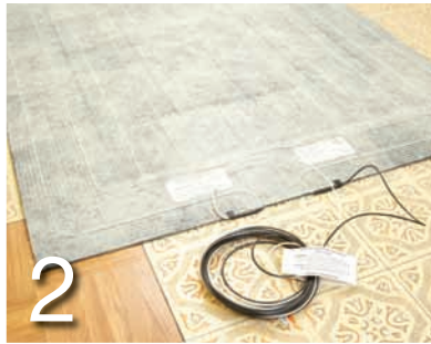
2 Lay out the heat mats so the lead wires are close to the thermostat.
