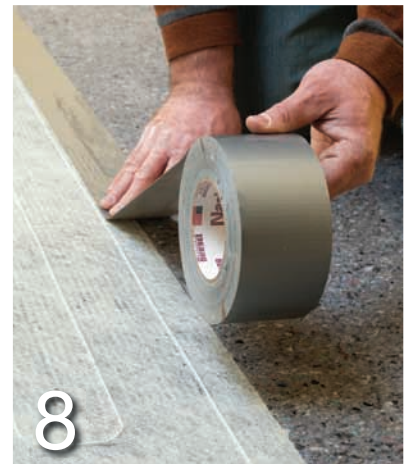
8 Using duct tape, secure underlayment adjacent to the heat mats.
