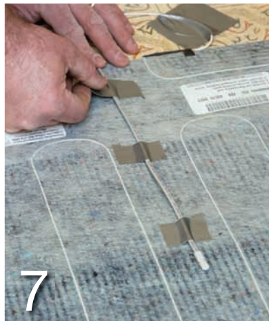
7 Install the heat sensor 8 in. from the end of the heat mat closest to the thermostat.
